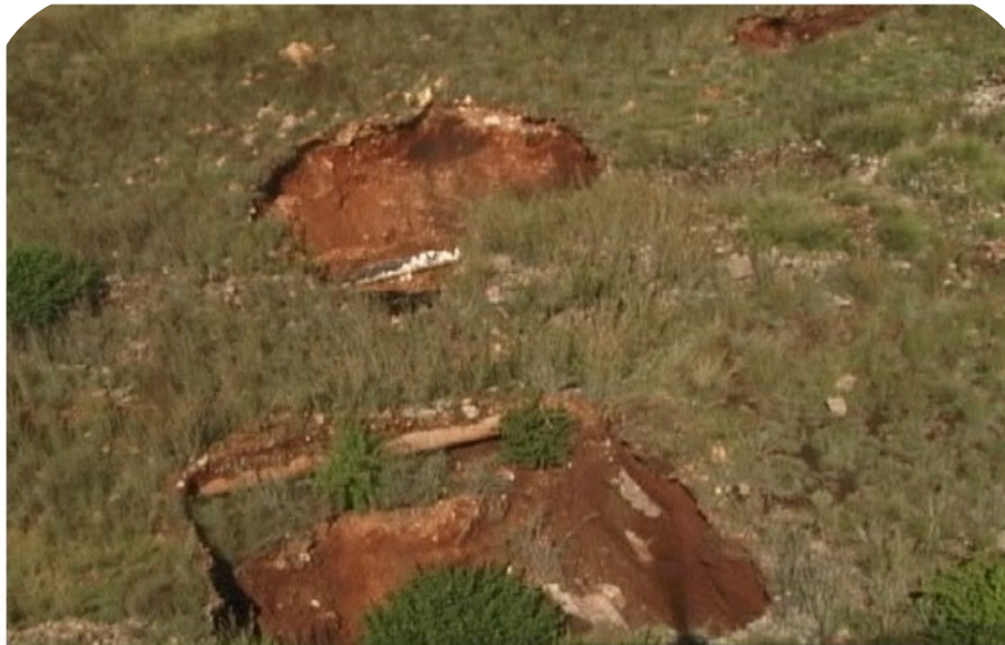
FIGURE 5: SINKHOLE AS RESULT OF LEAKING WATER MAINS
